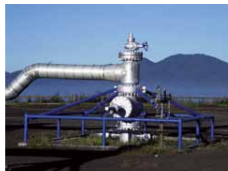
Chevron Geothermal Salak well head
