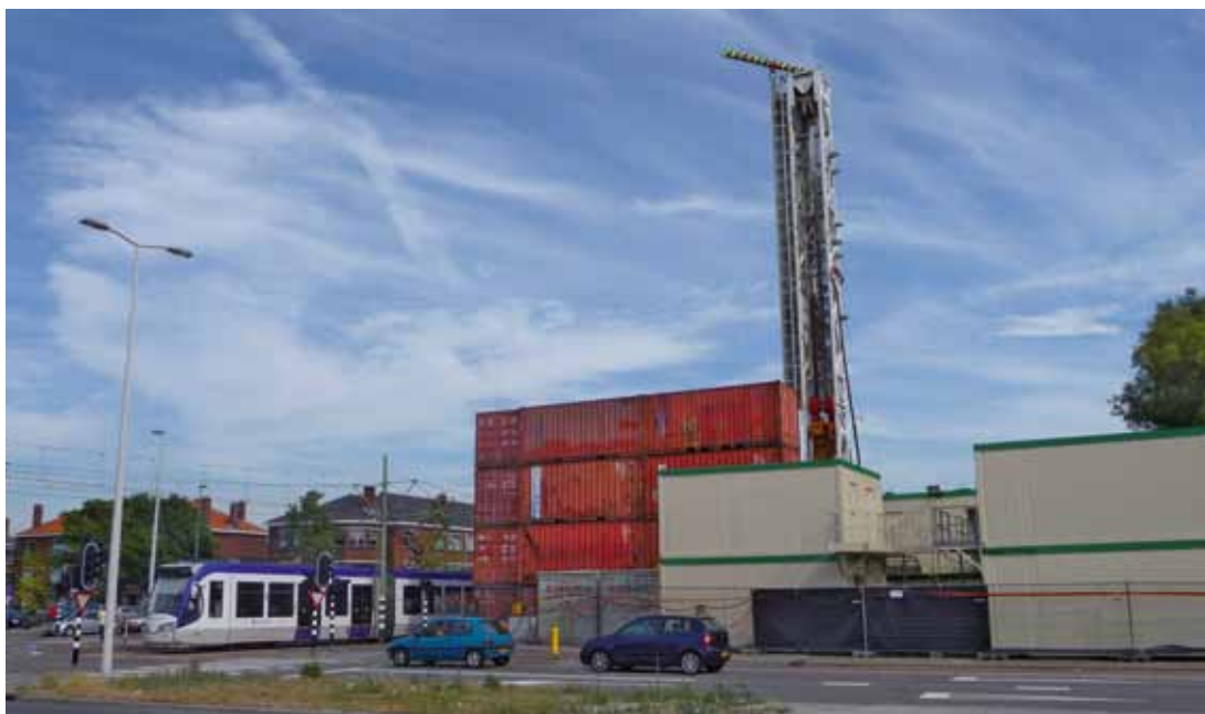
Drilling in The Hague (Netherlands) to a depth of 2km to reach temperatures that can be applied for electricity production
